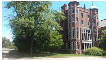
Cazenove Hall (Caz), 3 rd floor [relative address]
